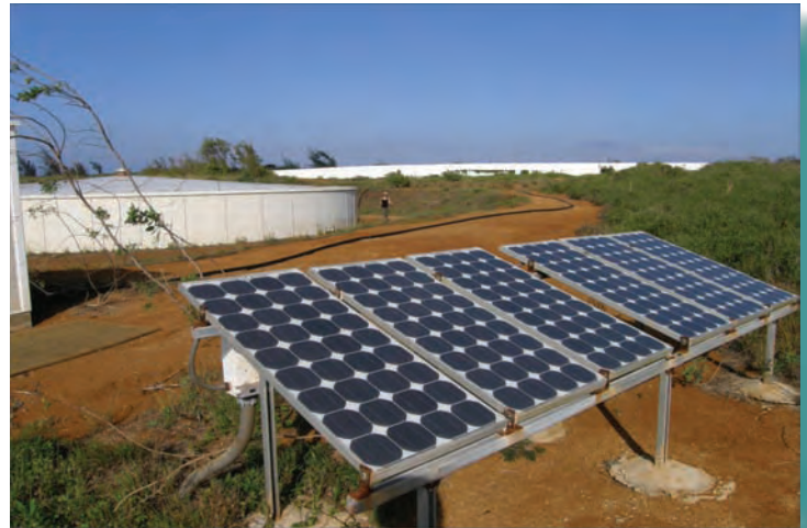
Photo-voltaic panels are used to power the pumps for our irrigation system. Even though they have proven to very effective, the initial investment was considerable.
