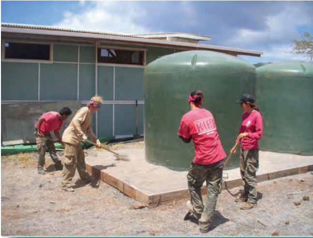
KIRC staff and volunteers complete the installation of water storage tanks that will collect the infrequent rainfall on island.
