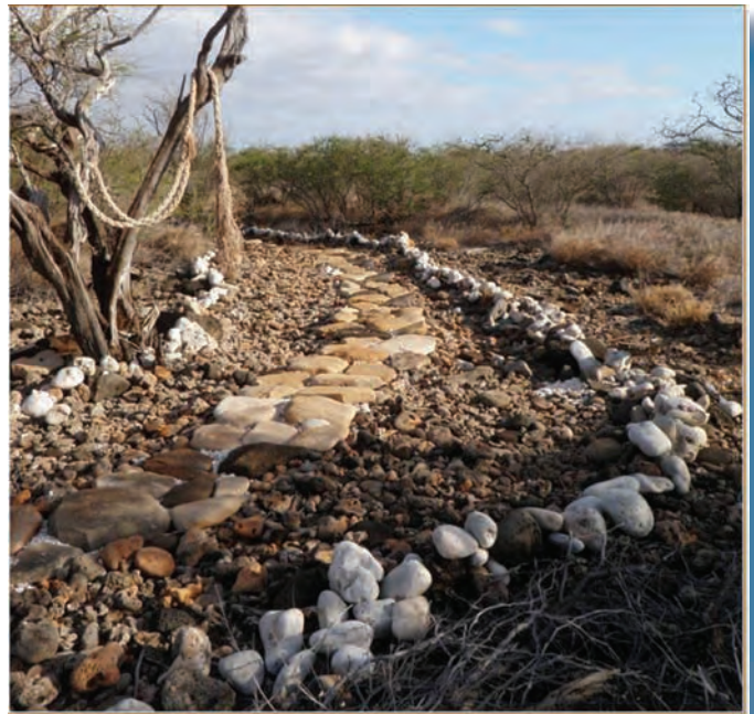
Volunteers help build a circum-island trail that will expand our cultural use of the island.
